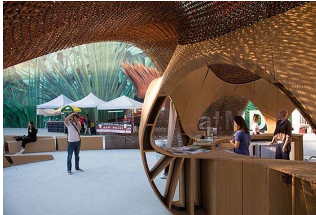
“Flotsam and Jetsam” structure designed by SHoP Architects for Design Miami and printed by Branch Technologies and Oak Ridge National Laboratories, courtesy of SHoP Architects
