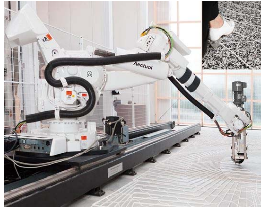
A robot printing elements of custom terrazzo flooring, courtesy of Aectual
