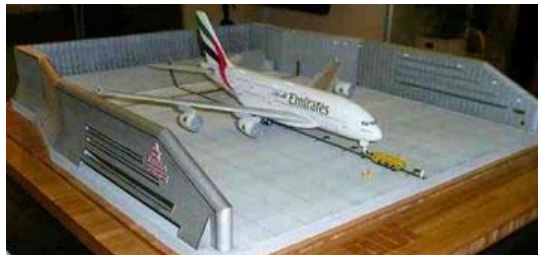
Model of engine ground test enclosure for Dubai airport, courtesy of LGM
